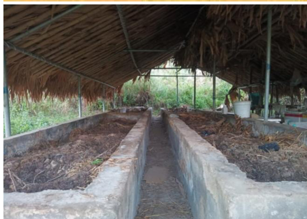
Fig. 3b. Vermi beds are made of brick masonry without the provision of vermiwash collection
