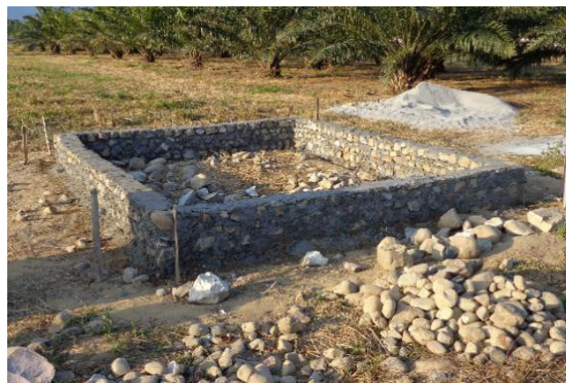
Fig. 1 a. NADEP tank construction
