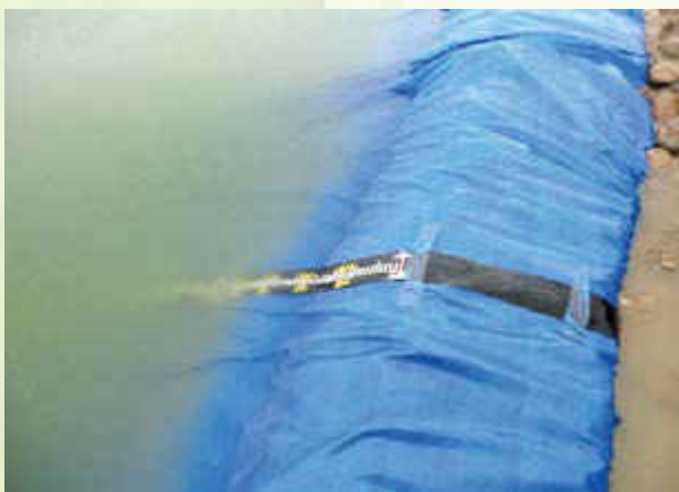
Fig. 8. Harvesting of in-situ rain water in the water harvesting pond
