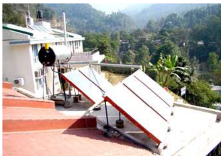
Fig. 2 Thermosyphon type flat plate collector solar water heater
